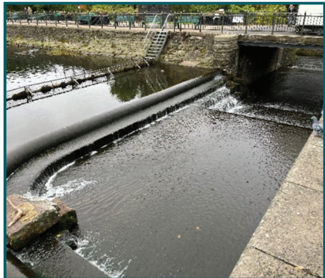
Photograph 2: Existing Roath Park spillway
